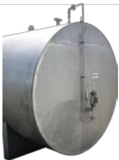
Dewater/sampling pump installed with anti-siphon valve for operation from ground level
